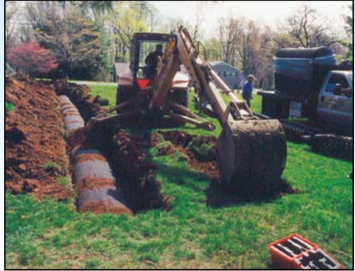
Trench installation demonstrating minimal disturbance of land.
