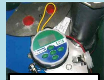
Pull controller up and out of chamber
