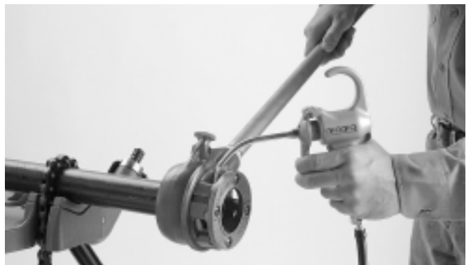
Figure 4 – Applying Thread Cutter Oil
