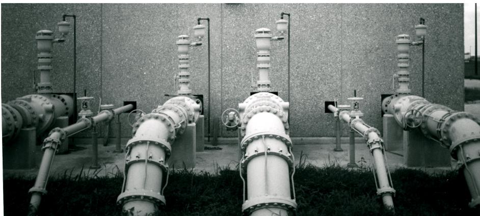
Surge-Suppression Air Valves and Isolation Valves in a pump discharge application.
