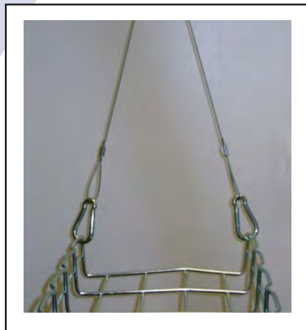
Cable Tray using Y-fit Karabiner
