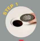
Secure shower drain to shower floor. Use silicone sealant for water tight seal.
