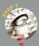
Tighten locking nut to secure shower drain to shower floor.
