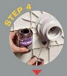
Apply solvent cement to secure shower drain and pipe.
