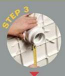
Measure distance from floor to stop inside of shower drain. Cut pipe to measured height.
