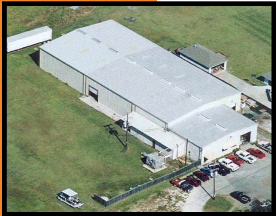
Manufacturing Plant Greenville, Texas
