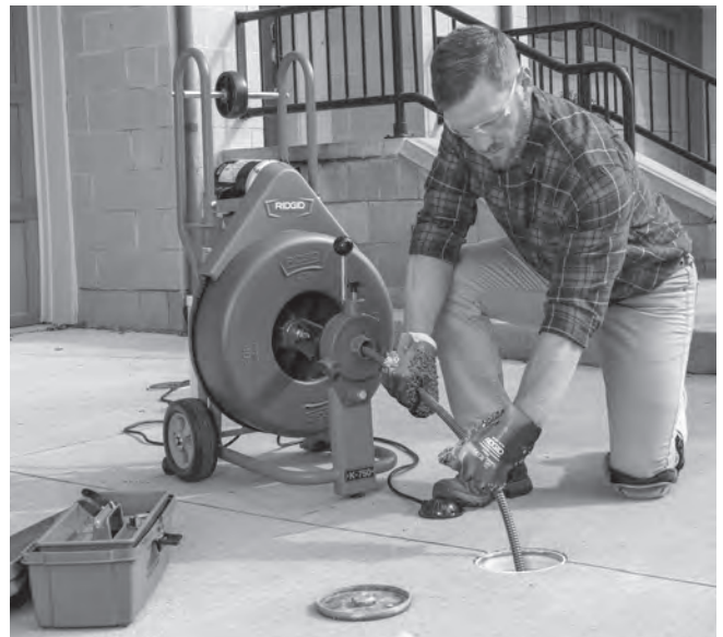
Figure 12 – In Operating Position, Manually Feeding Cable
