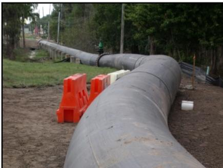
**DriscoPlex® 1000 pipe series** – These high density polyethylene (HDPE) PE4710/PE100 industrial pipes and fittings are produced in compliance with ASTM F714 and ASTM D3035 based on outside diameter pipe sizes. The product is a solid black HDPE pipe that meets ASTM D3350 Cell Classification of PE445574C and is suitable for a variety of industrial applications.
