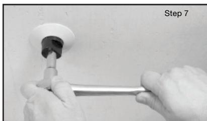
**Step 7.** Wrench-tighten the sprinkler using only the TYCO W-Type 25 Installation Wrench (Ref. Figure 3).
