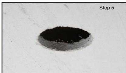
**Step 5.** Ensure that the ceiling/wall is smooth for the escutcheon to sit against and that the distance from the ceiling/wall surface to the sprinkler fitting is appropriate. As shown in Figures 5 and 6, the take-out dimensions are 1 inch for pendent sprinklers and 1-5/16 inches for horizontal sidewall sprinklers.
