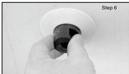
**Step 6.** With the escutcheon in place and with pipe-thread sealant applied to the pipe threads, hand-tighten the sprinkler into the sprinkler fitting using the TYCO W-Type 25 Installation Wrench with the wrench prongs fully engaged with the sprinkler wrenching notches. The wrench prongs are designed to engage the wrenching notches in the sprinkler body, and are also uniquely spaced to align with the sprinkler wrenching notches in one position.
