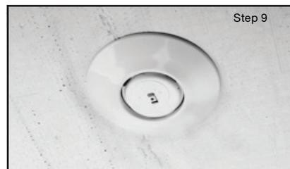
**Step 9.** After installation is complete, ensure that the RAVEN Escutcheon is held fast against the mounting surface and sits squarely against the ceiling around its entire perimeter.
