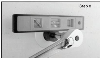
**Step 8.** For horizontal sidewall sprinklers, a Level can be placed on top of the flat surface of the TYCO W-Type 25 Installation Wrench to orient the sprinkler correctly.
