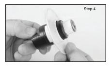
**Step 4.** With the Wrench on the sprinkler, place the escutcheon over the sprinkler.
