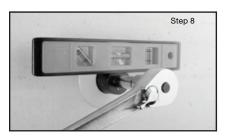
**Step 8.** For horizontal sidewall sprinklers, a Level can be placed on top of the flat surface of the TYCO W-Type 25 Installation Wrench to orient the sprinkler correctly.
