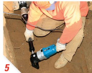
Make the tap, then reverse the process.
