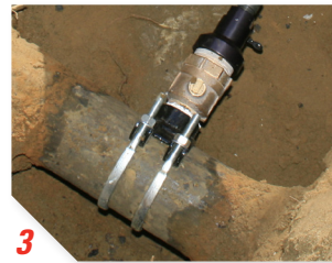
Turn independent feed until the pilot drill touches the pipe.
