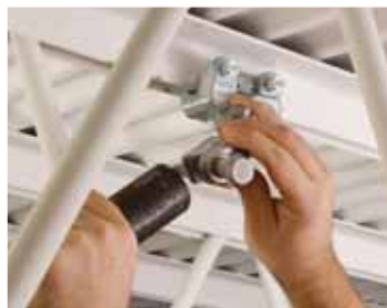
Step 1: Mount Universal Structural Attachment to chosen structural attachment (concrete, Bar Joist Adaptor, I-Beam Adaptor or other structural element).
