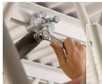
Step 2: Insert brace pipe and tighten shear bolt until head snaps off.
