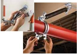
Step 1: Separate clamp and place around the pipe. Slide slotted component over bolt and tighten. Secure brace pipe by sliding clamp into pipe and snapping off bolt head.
