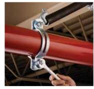
**Step 2:** Tighten nuts on the Easy Universal Sway Brace until securely locked in place.
