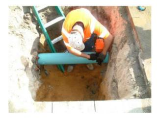
Apply AVT food grade tape to the pipe, wrapping the pipe 3 times making sure the tape is free of major wrinkles. This step allows the valve body to rotate and seal on the pipe with ease.
