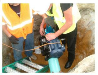
3. Rotate valve body down to one side until stop pin makes contact with ring.
