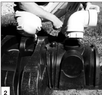
Insert Quick4 Plus Periscope.
