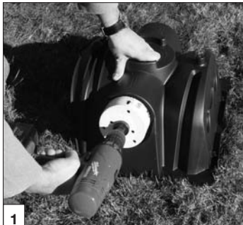
Drill endcap on side or top.
