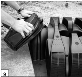
Place end cap outlet end.
