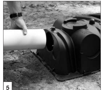
Insert inlet pipe.
