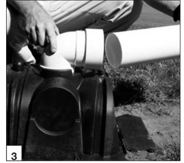
Connect inlet pipe.
