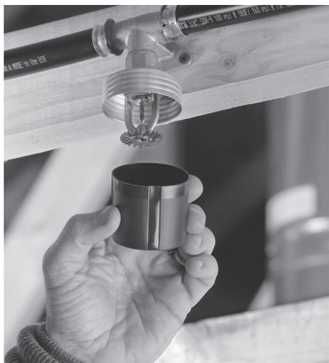
*Keep heads within protective shell during installation*
