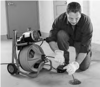
Figure 13 – In Operating Position, Manually Feeding Cable
