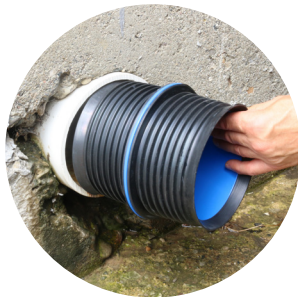
2) Lubricate gasket O.D. with soap & water solution
