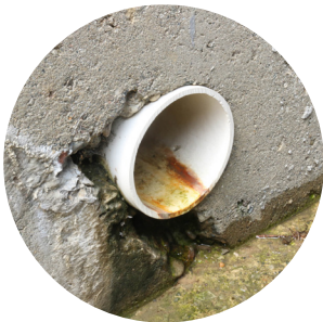
1) Clean and measure pipe I.D.
