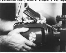
The conduit box cover is removed as shown prior to removing the motor for service. The wire nuts are removed and the flexible conduit connector is then removed.
