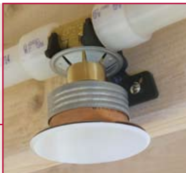
ProPEX Lead-free Brass Sprinkler Adapter in an AquaSAFE Looped Multipurpose System
