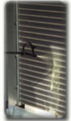
Shown above: An example of coil cleaning a microchannel with Triple-D®
