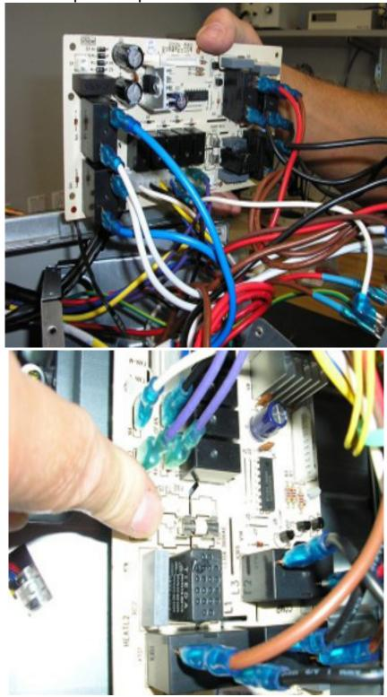
Figure 419 (Relay Board and Replaceable Fuse)
