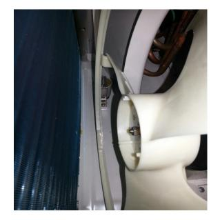
Figure 411 (Loosen Fan Shroud and Bellows Drain Valve Located inside Shroud)
