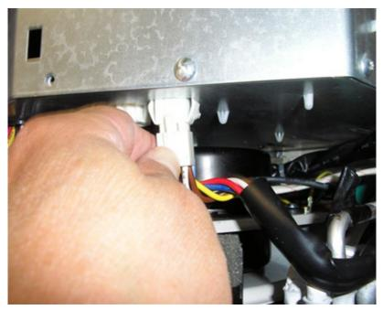
FIGURE 401 (Removal of Indoor Fan Wire Harness)
