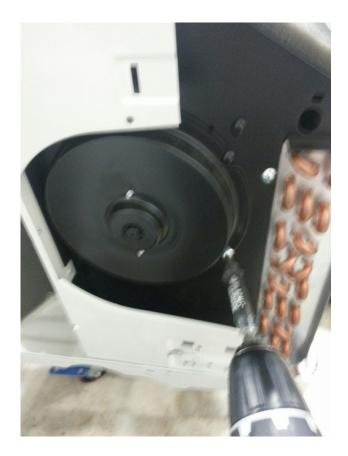
FIGURE 403 (Removal of Indoor Fan Grommet)
