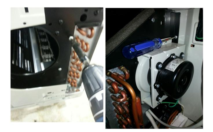
Figure 406 (Removal of Indoor Fan Housing Assembly)
