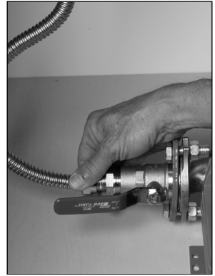
5. Connect flex lines to pump.
