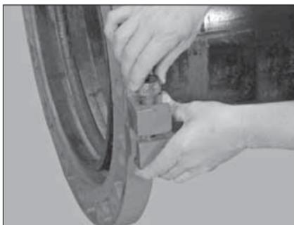
3. **ADD SECOND SEGMENT:** Add the second segment by inserting the draw bolts (provided) into the flange adapter with the nuts (provided) loosely and tightened uniformly. This will permit the flange adapter to be rotated for bolt hole alignment in later steps. Make sure the key of both segments engages completely in the groove.
