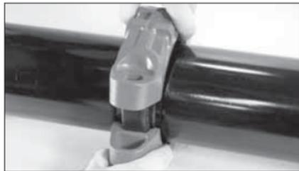
2. **INSTALL HOUSINGS:** Install the housings over the gasket. Make sure the housings' keys engage the grooves completely on both pipe ends. Refer to the notice above for Styles 475/475DX Couplings.
