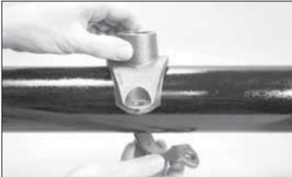
**3. INSTALL HOUSINGS:** Install the outlet housing onto the pipe by centering the locating collar in the hole. To check for proper engagement, slide the outlet housing back and forth while pushing down. A properly positioned outlet housing can be moved only a small amount in any direction.
