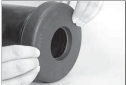
**3. INSTALL GASKET:** Install the larger opening of the gasket over the larger pipe end. Make sure no portion of the gasket extends into the pipe groove.
