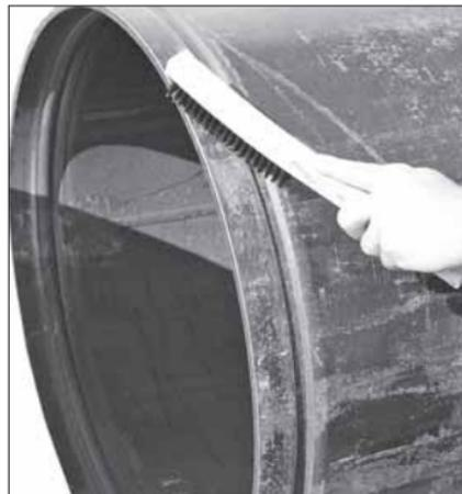
1b. Clean the outside surface of the pipe, from the groove to the pipe end, to remove all oil, grease, loose paint, and dirt.
