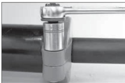
**7. TIGHTEN NUTS:** Tighten the nuts evenly by alternating sides until metal-to-metal contact occurs at the bolt pads. Make sure the housings' keys engage the grooves completely. **NOTE:** It is important to tighten the nuts evenly to prevent gasket pinching.
