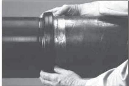
**4. JOIN PIPE ENDS:** Align and bring the NPS and JIS pipe ends together. Slide the gasket into position and center it between the groove in each pipe end.
