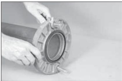
5b. When the bolt holes are aligned, insert a standard, full-shank diameter assembly bolt through the other mating hole of the Vic-Flange Adapter.
