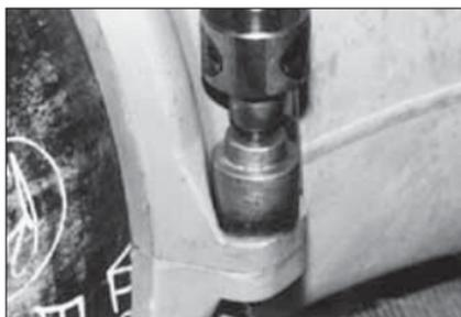
**4. TIGHTEN NUTS:** Tighten all nuts evenly by alternating sides until metal-to-metal contact occurs at the bolt pads. Make sure the housings' keys engage the grooves completely. **NOTE:** It is important to tighten all nuts evenly to prevent gasket pinching.
