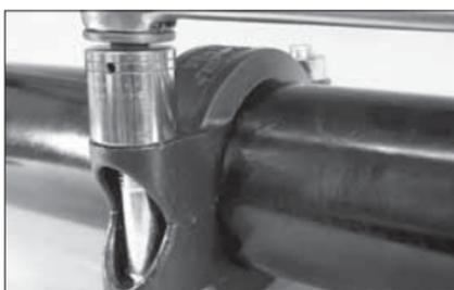
**7. TIGHTEN NUTS:** Tighten the nuts evenly by alternating sides until metal-to-metal contact occurs at the bolt pads. Make sure the housings' keys engage the grooves completely. **NOTE:** It is important to tighten the nuts evenly to prevent gasket pinching.
