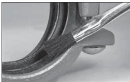
**4. LUBRICATE GASKET:** Apply a thin coat of Victaulic Lubricant or silicone lubricant only to the sealing lips of the gasket interior. **NOTE:** The gasket exterior is supplied with a factory-applied lubricant, so there is no need to remove the gasket from the housings to apply additional lubricant to the exterior surface.
