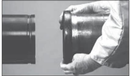
**3. INSTALL GASKET:** Install the larger opening of the gasket (marked NPS) over the larger pipe end (NPS side). Make sure the gasket does not overhang the pipe end.
