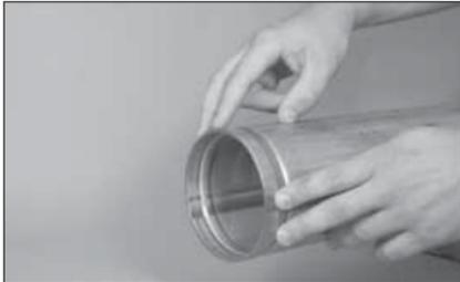
**1. CHECK PIPE ENDS:** The outside surface of the pipe, between the groove and the pipe end, must be smooth and free from indentations, projections (including weld seams), and roll marks to ensure a leak-tight seal. All oil, grease, loose paint, dirt, and cutting particles must be removed.
