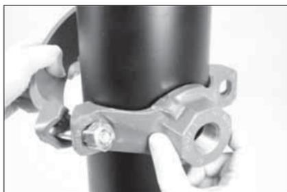
**3. INSTALL HOUSINGS:** Rotate the lower housing so that it is positioned approximately 90° to the upper (outlet) housing, as shown above. Place the upper (outlet) housing onto the face of the pipe in line with the outlet hole cut into the pipe. Rotate the lower housing around the pipe.
