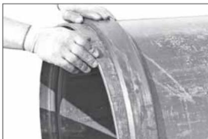
3. **POSITION GASKET:** Position the gasket over the pipe end or AGS Vic-Ring. Make sure the gasket does not overhang the pipe end or AGS Vic-Ring.
