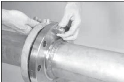
7. THREAD NUTS ONTO MATING BOLTS: Thread a nut onto each mating bolt. Tighten the nuts until they are finger-tight.
