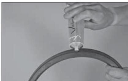
2. **CHECK GASKET AND LUBRICATE:** Check the gasket to make sure it is suitable for the intended service. The color code identifies the gasket grade. Apply a thin coat of Victaulic lubricant or silicone lubricant to the gasket lips and exterior.
