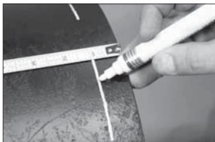
**2. MARK PIPE ENDS:** Using a measuring tape and a bright-colored pencil or paint stick, place a mark 1 inch/25mm from the pipe ends. This mark will be used for reference in centering the gasket during installation. Make at least four of these marks equally-spaced around the circumference of the pipe ends.
