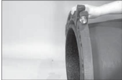
**3. ADD ADDITIONAL SEGMENTS:** Add each segment by inserting the draw bolts (provided) into the flange adapter with the nuts (provided) loosely and uniformly tightened. This will permit the flange adapter to be rotated for bolt hole alignment in later steps.
