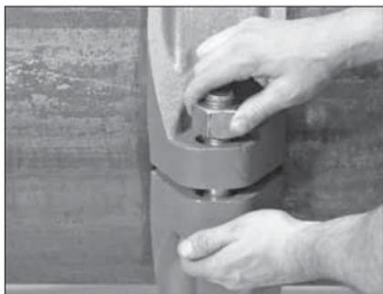
**6. INSTALL HOUSINGS:** Install the housings over the gasket. Make sure the housings' keys engage the groove completely in each pipe end or AGS Vic-Ring. Support the segments while preparing to install the bolts and nuts.
