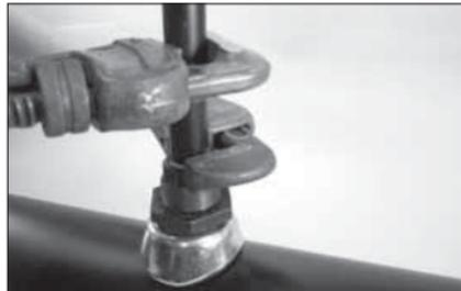
**9. MAKE CONNECTION:** Make the required connection by using a second wrench on the top hex only. To prevent loosening of the outlet in the hole, **DO NOT** use the assembly nut for tightening this connection.
