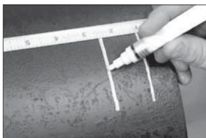
**2a.** Refer to the “Insertion Depth Requirements” table below. Using a measuring tape and a bright-colored marking pencil or paint stick, make an additional mark on the pipe ends at the measurement listed in this table. This mark will be used for visual inspection to make sure the pipe is inserted properly in the coupling. Make at least four of these marks equally-spaced around the circumference of the pipe ends.
