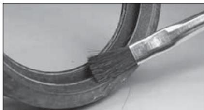
3. **LUBRICATE GASKET:** Apply a thin coat of Victaulic Lubricant or silicone lubricant to the gasket sealing lips and exterior. It is normal for the gasket surface to have a hazy white appearance after it has been in service. **NOTE: HOUSINGS AND GASKETS FOR 107H COUPLINGS ARE NOT INTERCHANGEABLE WITH HOUSINGS AND GASKETS FOR 107 COUPLINGS.**
