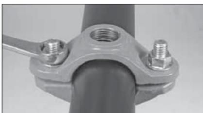
**5. TIGHTEN FLANGE NUTS:** Tighten the flange nuts evenly to an approximate torque value of 20ft-lbs/27.1-N•m to ensure proper gasket compression. **NOTE:** To avoid over-tightening the flange nuts, use a wrench with a maximum length of 8 inches/200mm. **DO NOT** over-tighten the flange nuts.
