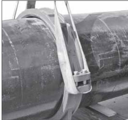
**6. INSTALL HOUSINGS:** Using a strapping method, similar to the one shown in the photos above with the bolts installed in the bolt holes, install the housings over the gasket. Make sure the housings' keys engage the groove completely in each pipe end or AGS Vic-Ring.
