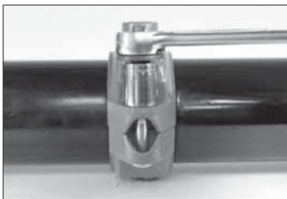
**8. TIGHTEN NUTS:** Tighten the nuts evenly by alternating sides until metal-to-metal contact occurs at the bolt pads. Make sure the housings' keys engage the grooves completely. **NOTE:** It is important to tighten the nuts evenly to prevent gasket pinching.
