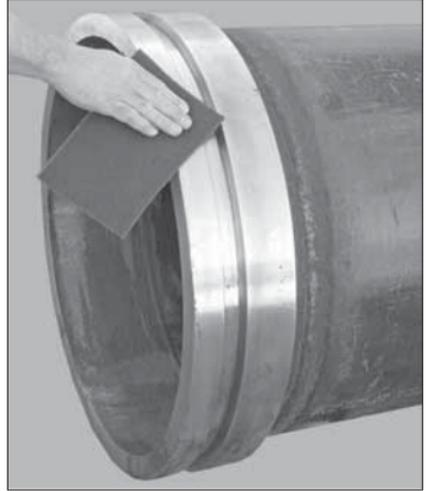
**1.** Prior to welding a Vic-Ring onto the pipe end, weld seams must be ground flush to the pipe surface (outside diameter). Grind the weld seam from the pipe end to a minimum distance of 6 inches/152 mm back from the pipe end. This area must be smooth and free from indentations, projections, and roll marks.
