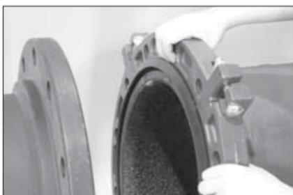
**6. ALIGN VIC-FLANGE AND MATING FLANGE:** Rotate the Vic-Flange on the pipe end, as required, to align the holes with the mating flange.
