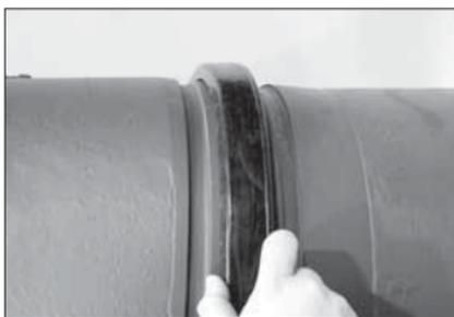
**4a. If the gasket was turned inside out in step 3a for larger size (non-AGS) couplings:** Roll the gasket into position and center it between the groove in each pipe end. Make sure no portion of the gasket extends into the groove in either pipe end.
