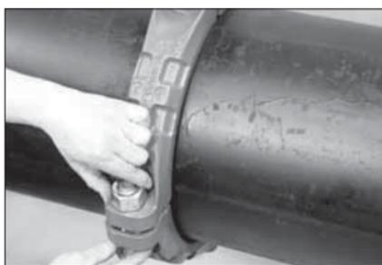
**3a. INSTALL REMAINING SEGMENT ASSEMBLY:** Install the second assembly onto the pipe. Make sure the housings' keys engage the grooves completely on both pipe ends. While supporting the weight of the assembly, install the remaining bolts, and thread the nuts finger-tight onto the bolts. **NOTE:** Make sure the oval neck of each bolt seats properly in the bolt hole.
