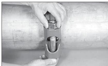
2. **INSTALL HOUSINGS:** Install the housings over the gasket with the tongue and recess features mated
