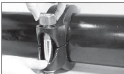
**6. INSTALL BOLTS/NUTS:** Install the bolts, and thread a nut finger-tight onto each bolt. **NOTE:** Make sure the oval neck of each bolt seats properly in the bolt hole.
