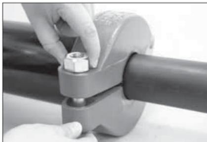
**6. INSTALL BOLTS/NUTS:** Install the bolts, and thread a nut finger-tight onto each bolt. **NOTE:** Make sure the oval neck of each bolt seats properly in the bolt hole.
