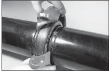
7. **INSTALL HOUSINGS:** Install the housings over the gasket. Make sure the housings' keys engage the grooves properly on both pipes/mating components.
