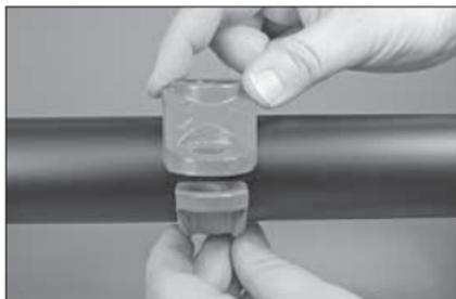
**3. INSTALL HOUSINGS:** Install the outlet housing onto the pipe by centering the locating collar in the hole. To check for proper engagement, slide the outlet housing back and forth while pushing down. A properly positioned outlet housing can be moved only a small amount in any direction.
