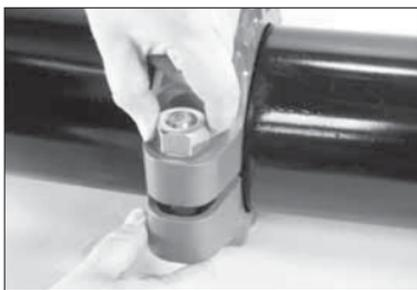
3. **INSTALL BOLTS/NUTS:** Install the bolts, and thread a nut finger-tight onto each bolt. For couplings supplied with stainless steel hardware, apply an anti-seize compound to the bolt threads. **NOTE:** Make sure the oval neck of each bolt seats properly in the bolt hole.
