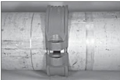
**6. INSTALL HOUSINGS:** Install the housings over the gasket. Make sure the housings' keys engage the groove completely in each pipe end or AGS Vic-Ring. Support the segments while preparing to install the bolts and nuts.
