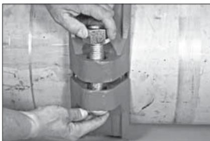
**7. INSTALL BOLTS/NUTS:** Install the bolts, and thread a nut finger-tight onto each bolt. **NOTE:** Make sure the oval neck of each bolt seats properly in the bolt hole.
