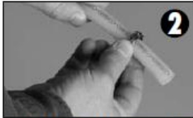
2 Slide clamp or crimp ring over tube.
