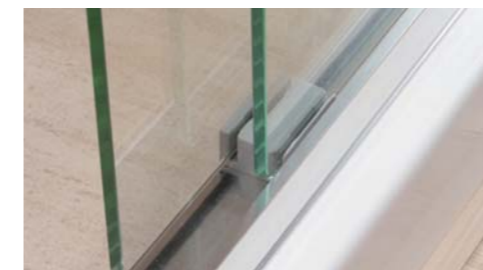
Flat tracks at the bottom prevents water accumulation for ease of cleaning and enhanced hygiene.
