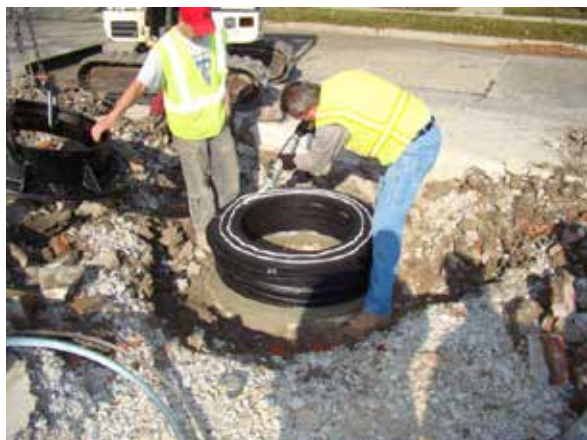
11. Place two ½" beads of M-1 adhesive on the top surface of the Finish or Angle Ring prior to setting the manhole frame casting.
