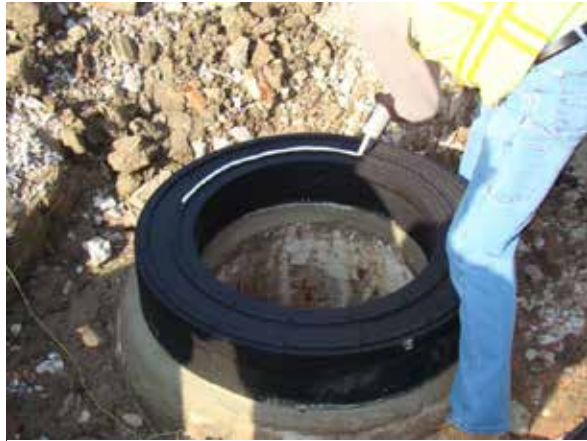
7. If multiple Grade Rings are required, repeat step 6 until all Grade Rings have been properly installed and then proceed to step 8.
