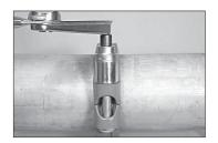
4. TIGHTEN NUTS: Tighten all nuts evenly by alternating sides. Make sure the housings' keys engage the grooves completely on both pipe ends. Apply torque to each nut with a torque wrench. Refer to the following table for the torque requirement. NOTE: It is important to tighten the nuts evenly to prevent gasket pinching.
