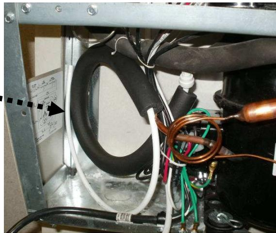
For split level “Versafiller ready” coolers, the tube to plumb in the Versafiller is packaged in the dummy unit.
