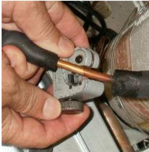
4. Install TEE fitting by connecting the copper tubing to each end. Then install the 32" piece of plastic tubing to the TEE branch.
