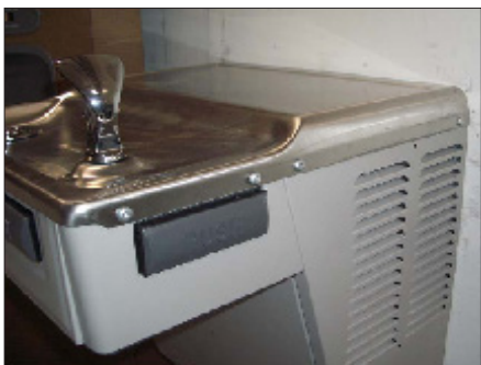
Remove Basin Fasteners
