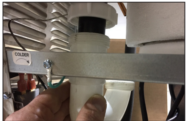
Reattach drain line to P-trap
