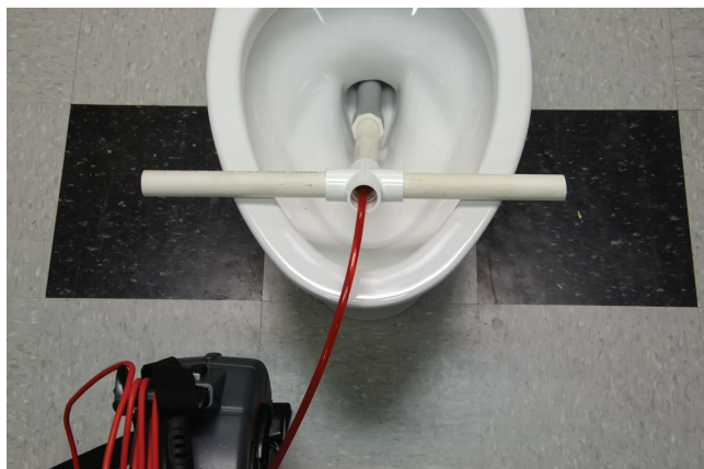
Figure 23 – Using a PVC Guide Tube
