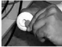
**Step C** – Cut the blue tubing between the RO faucet and the RO module at a desired location to splice in the in-line final filter.
