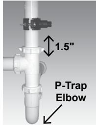
**Step D** – Assemble the drain saddle around the drain pipe and align drain saddle fitting opening with the hole drilled in the previous step - you may use a small screwdriver to feed through the drain saddle into the drain pipe to aid with the alignment. Using a Phillips screw driver tighten the drain saddle bolts evenly and securely on both sides.
