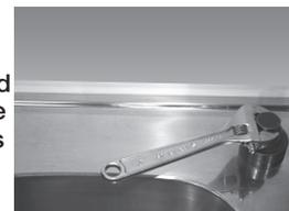
**Step A** – Drill a ¼" pilot hole. Use a ½" Hole Punch and an adjustable wrench to punch the hole in the sink. Change to the 1¼" Hole Punch to enlarge the hole
