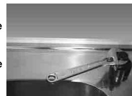
**Step A** – Drill a 1/4" pilot hole. Use a 1/2" Hole Punch and an adjustable wrench to punch the hole in the sink.
