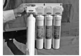
**Step D** – Repeat this procedure for the 2nd filter cartridges. When finished, flush your tank completely once to remove any natural carbon fines from the UF Drinking system. Check over the next 24 hours to ensure no leaks are present.
