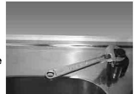
**Step A** – Drill a ¼" pilot hole. Use a ½" Hole Punch and an adjustable wrench to punch the hole in the sink. Change to the 1¼" Hole Punch to enlarge the hole
