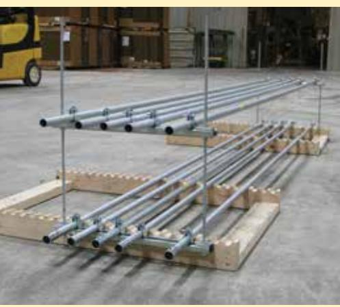
The spacing between conduits across the channel needs to be the same so that they meet up with each other when the individual runs are installed. It is recommended that installers use custom wooden jigs with notches at the spacing for each piece. They can be easily made on the jobsite with pieces of wood and customized for individual situations.
