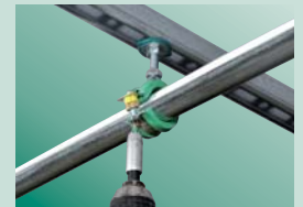
Final tighten assembled clamp
