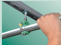
Place reinforced pipe into clamp
