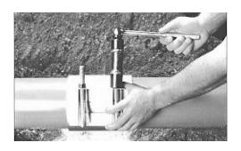
Tighten the nuts evenly with a hand wrench to the following torque values. *Trick of the Trade: Pneumatic wrenches could cause the stainless nuts to seize on the stainless steel studs.*
