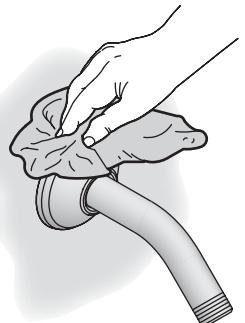
Remove the excess sealant.
