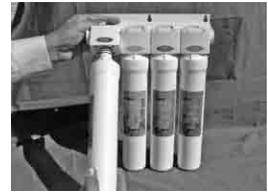
**Step D** – Repeat this procedure for the 2nd filter cartridges. When finished, flush your tank completely once to remove any natural carbon fines from the RO system. Check over the next 24 hours to ensure no leaks are present.
