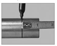
1. When using a ruler or tape measure, refer to the "Vic-Press Schedule 10S Insertion Depth Requirements" table below. Measure back from the pipe end. Place a mark around the pipe circumference with a marker or paint stick, as shown above.
