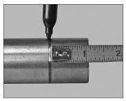
1. Refer to the "Vic-Press Schedule 10S Slip Coupling Minimum Insertion Depth Requirements" table below. Use a ruler or tape measure to measure back from the pipe end. Place a mark around the pipe circumference with a marker or paint stick, as shown above.
