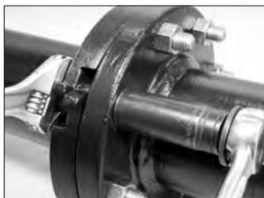
**9. TIGHTEN NUTS:** Tighten all nuts evenly in the applicable pattern shown above until metal-to-metal contact is achieved between the flange faces or the flange-bolt torque requirement for the mating flange is achieved.
