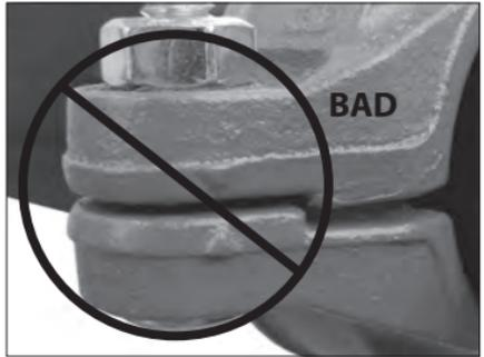
Visually inspect the bolt pad location at every joint to verify that metal-to-metal contact is achieved around the bolt pad perimeter (approximately between the two sets of indicator arrows).
