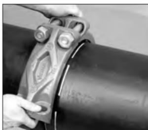
**9a. INSTALL FIRST PRE-ASSEMBLED HALF:** Install the first pre-assembled half over the gasket.
