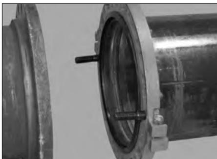
**8. INSTALL STANDARD FULL-SHANK-DIAMETER ASSEMBLY BOLTS AT LAP JOINTS:** Install a standard full-shank-diameter assembly bolt into each of the lap-joint bolt holes. Refer to the “Helpful Information” table on page 234 for the required assembly bolt size and length.
