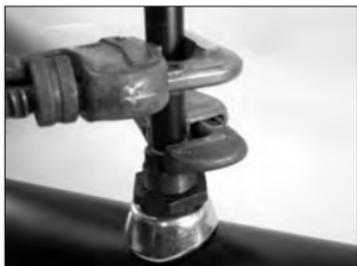
**9. MAKE CONNECTION:** Make the required connection by using a second wrench on the top hex only. To prevent loosening of the outlet in the outlet hole, **DO NOT** use the assembly nut for tightening this connection.
