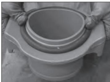
**5b. INSTALL O-RING:** Press the o-ring into the groove on the underside of the spigot housing. **DO NOT** place the o-ring on the pipe and then attempt to push the locating collar through it. This may push the o-ring into the outlet hole, and will prevent proper sealing.
