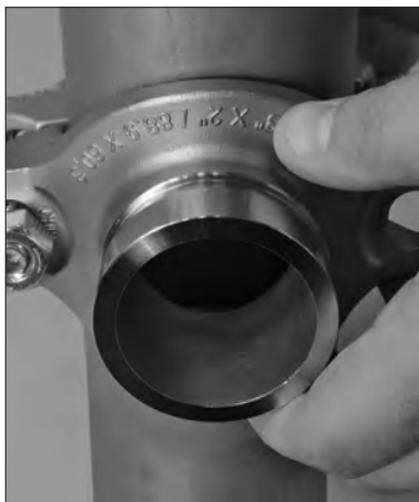
**4. INSTALL HOUSINGS:** Rotate the lower housing so that it is positioned approximately 90° to the upper (outlet) housing, as shown above. The upper (outlet) housing’s locating collar shall be placed into the outlet hole. Rotate the lower housing around the pipe.
