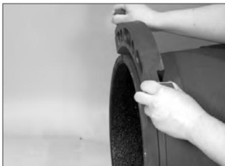
**2. INSTALL FIRST SEGMENT:** Install the first segment onto the pipe. Verify that the segment's key section completely engages the groove. **NOTE:** On vertical pipe, the segments shall be supported in place until all segments are installed and fastened together. For horizontal pipe, the first segment can be balanced on top of the pipe, as shown to the left.
