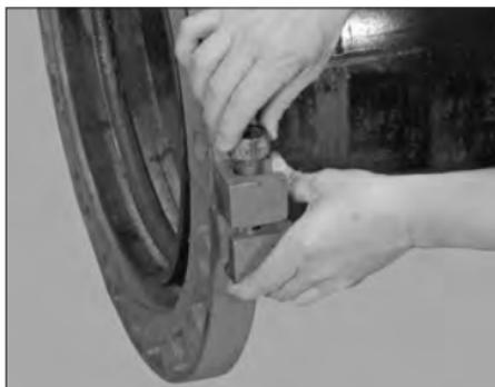
**3. INSTALL SECOND SEGMENT:** Install the second segment onto the pipe. Install the provided draw bolts into the Style W741, as shown to the left. Thread a provided nut loosely onto each draw bolt. **NOTE:** The nut should be installed at least flush with the end of the draw bolt but loose enough to permit rotation of the Style W741 for bolt hole alignment in later steps. Verify that the key section of both segments completely engages the groove.
