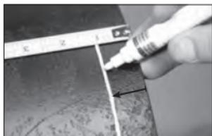
**3a. PLACE GASKET-CENTERING MARK ON PIPE/FITTING ENDS:** Using a measuring tape and a bright-colored pencil or paint stick, place a mark 1 inch/25 mm from the pipe/fitting ends. This mark will be used for reference in centering the gasket during installation. Make at least four marks, equally spaced around the circumference of the pipe/fitting ends.
