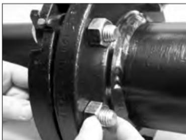
**8. INSTALL REMAINING STANDARD FULL-SHANK-DIAMETER ASSEMBLY BOLT/NUTS:** Insert a standard full-shank diameter assembly bolt through each remaining hole in the Style 741, 841, 743, or 744 and mating flange. Tighten a nut onto each bolt.
