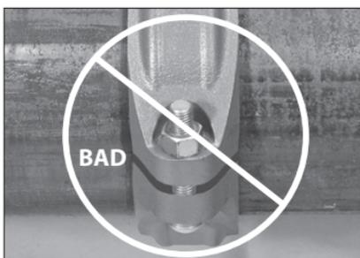
8. Visually inspect each bolt pad location at every joint to verify that metal-to-metal contact is achieved across the entire bolt pad section.
