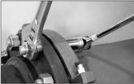
**10b. TORQUE ALL STANDARD FULL-SHANK-DIAMETER ASSEMBLY BOLTS:**
