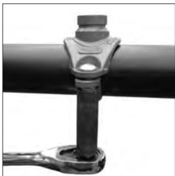
**5. TIGHTEN FLANGE NUTS:** Verify that the locating collar is still positioned properly in the outlet hole. Tighten the flange nuts evenly by alternating sides, maintaining nearly uniform bolt pad gaps, to a maximum torque value listed below to ensure proper gasket compression. Verify that the oval neck of each bolt seats properly in the bolt holes. Refer to the “Helpful Information” table below.
