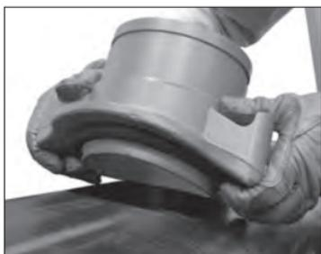
**6. PLACE HOUSING:** Place the housing by inserting the locating collar into the outlet hole in the pipe. Verify that the o-ring remains in the groove on the housing and does not fall into the outlet hole.
