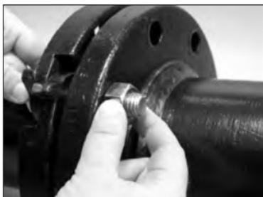
**7. JOIN STYLE 741, 841, 743, OR 744 AND MATING FLANGE:** Insert the assembly bolts, installed in step 7b, into the mating flange holes. Tighten a nut onto each bolt to prevent the bolts from pulling out.
