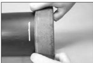
**6. INSTALL GASKET:** Install the gasket over the pipe/fitting end. **NOTE:** Verify that the gasket does not overhang the pipe/fitting end.
