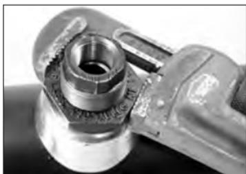
**7. WRENCH-TIGHTEN ASSEMBLY NUT:** Wrench-tighten the assembly nut until the collar deforms and contacts the pipe evenly on all sides. Maintain collar/gasket alignment to prevent gasket pinching.
