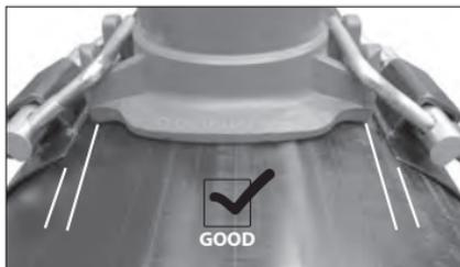
**11. INSPECT ASSEMBLY GAPS:** Verify that the spigot housing is an equal distance from the strap on each side. If the strap hardware does not grip the housing evenly from both sides, the assembly may be pulled out of alignment, causing the housing to angle into the outlet hole and creating improper compression of the o-ring.
