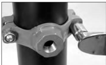
**7. TIGHTEN NUTS:** Verify that the locating collar is still positioned properly in the outlet hole. Using an impact tool or a standard socket wrench with a deep-well socket, tighten the nuts evenly by alternating sides, maintaining nearly uniform bolt pad gaps, until the upper (outlet) housing contacts the pipe completely. Verify that the oval neck of each bolt seats properly in the bolt holes.
