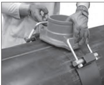
**8. ATTACH STRAP:** On the opposite side of the pipe, pull the second U-bolt up and hook it over the second retaining gusset of the spigot housing. **NOTE:** If there is inadequate length to perform this step, loosen the nuts on the U-bolts to lengthen the assembly.
