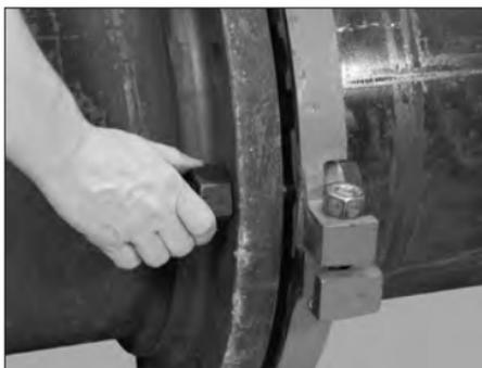
**9. JOIN W741 AND MATING FLANGE:** Direct the assembly bolts, installed in step 8, into the mating flange holes. Tighten a nut onto each bolt to prevent the bolts from pulling out.
