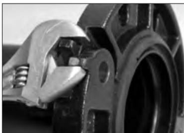
**6a. FOR STYLE 741, 841, AND STYLE 744 ONLY:** Closure lugs are provided for ease of installation. Clamp both lugs with a wrench or pliers to bring the lap-joint bolt holes into alignment.
