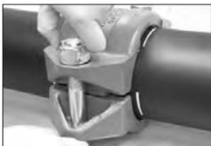
**9. INSTALL BOLTS/NUTS:** Install the bolts, and thread a nut finger-tight onto each bolt.
