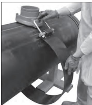
**7. PLACE STRAP:** Push one end of the strap underneath the pipe and hook one U-bolt over the retaining gusset of the spigot housing.
