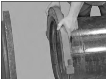
**2. INSTALL FIRST SEGMENT:** Install the first segment onto the pipe. Verify that the segment's key section completely engages the groove. **NOTE:** On vertical pipe, the first segment shall be supported in place until the second segment is installed and fastened to the first segment. For horizontal pipe, the first segment can be balanced on top of the pipe, as shown to the left.
