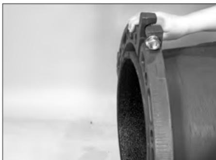
**3. INSTALL ADDITIONAL SEGMENTS:** Install each segment onto the pipe. Install the provided draw bolts into the Style 741, as shown to the left. Thread a provided nut loosely onto each draw bolt. **NOTE:** The nut should be installed at least flush with the end of the draw bolt but loose enough to permit rotation of the Style 741 for bolt hole alignment in later steps. Verify that the key section of all segments completely engages the groove.
