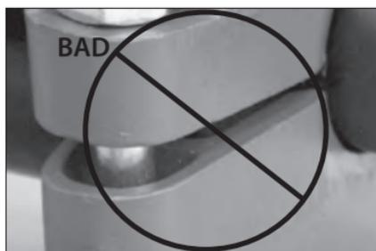
7. Visually inspect each bolt pad location at every joint to verify that metal-to-metal contact is achieved across the entire bolt pad section.
