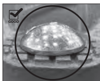
OVAL NECK OF BOLT SEATED PROPERLY
