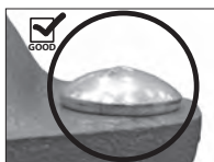
OVAL NECK OF BOLT SEATED PROPERLY
