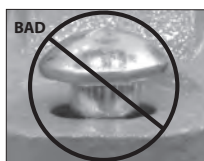
OVAL NECK OF BOLT NOT SEATED PROPERLY
