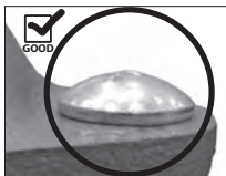
OVAL NECK OF BOLT SEATED PROPERLY
