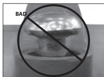
OVAL NECK OF BOLT NOT SEATED PROPERLY
