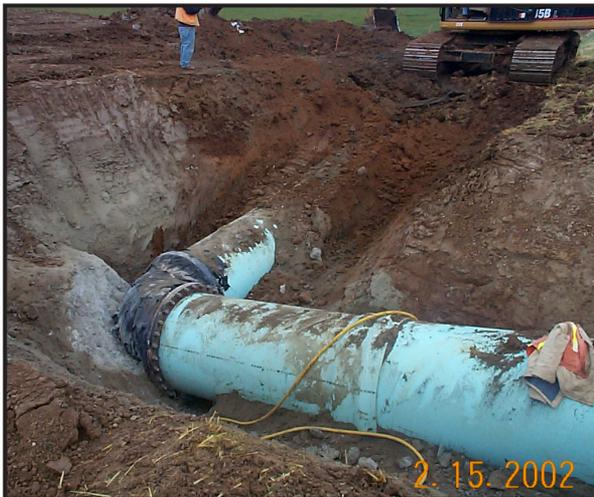
**Foundation:** An adequate or stable foundation should be present (or provided) to uniformly support the full length of the pipe. Bell holes should be provided at each joint to permit proper assembly and support of the pipe. Unstable trench bottoms shall be stabilized by methods and with materials required, by the specifying engineer, to provide adequate and permanent support for the conditions encountered.
