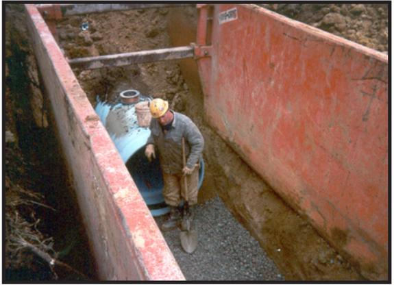
The bedding should consist of an evenly graded, free flowing, granular material which is free of large stones or frozen material and with particle size of up to approximately 10% of the pipe size and no larger than 1 1/2" in size. Bell holes should be utilized to reduce axial deflection and support the barrel of the pipe.
