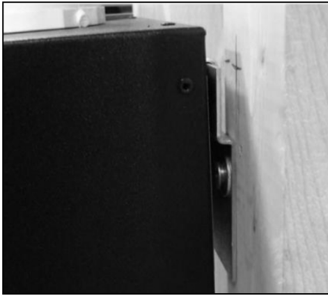
Figure 2 - Boiler Mounted to Mounting Bracket on Pallet
