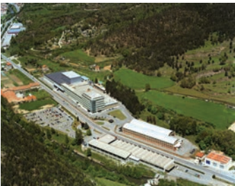
Ripoll Factory (Spain)
