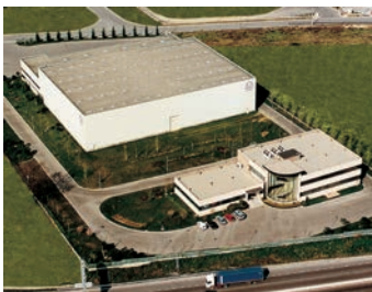
Logistics Center in Parets (Spain)
