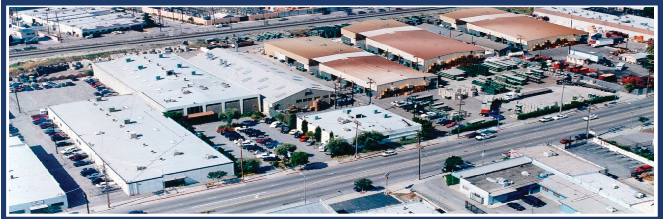
Corporate Facility / North Hollywood, California
