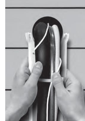
(4) Run lineset, drain hose, wiring etc. over the fitting and duct bases and secure to duct clips using tie wraps of sufficient size.
