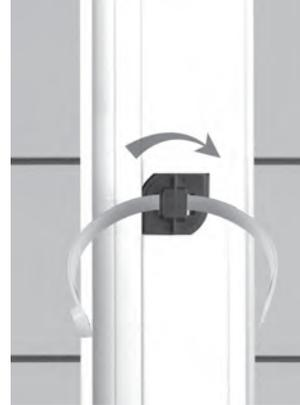
(3) Position and twist in lineset duct clips (Model# LDC) evenly spaced throughout installation. Nylon cable ties (not included) slip through lineset duct clips and fasten around lineset.
