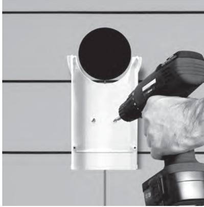
(1) Determine the path which the lineset will follow and strike a chalk line to mark the surface material. Attach the base only of all fittings first (ducting will be placed last), along the marked path, using fasteners of sufficient length (not provided). Pre-drill where necessary. Duct must terminate **with a fitting to prevent cover** from sliding out of position.
