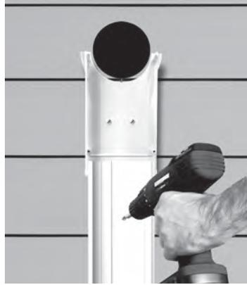
(2) Once all fitting bases are secured to the siding, measure and cut LD Ducting to fit as needed. Remember to account for some seasonal expansion and contraction. Install and fasten LD Ducting bases. Attach bases only to structure through provided punch outs using fasteners of sufficient length (not provided).
