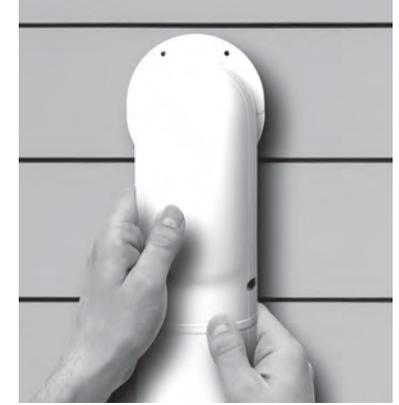
(5) Snap straight duct top over mating straight base pieces. Seat fitting tops over mating fitting bases and secure with provided stainless screws. Duct **must** terminate with a fitting to prevent cover from sliding out of position. If duct is to be painted, or duct is a dark color, adhere cover to base with pvc cement.
