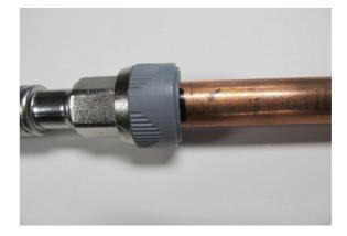
4. Insert the pipe into the fitting up to the 1.2" mark. Pull on the pipe to make sure that it is secure. Test the system for leakage before use.
